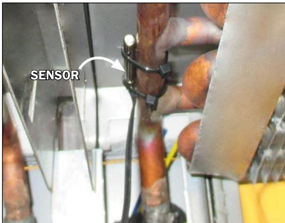
**Fig. 4 Gravity coil sensor**
