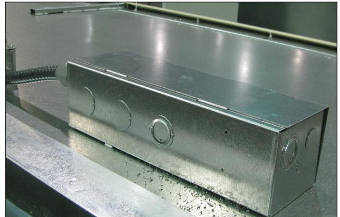
Fig. 14 Junction box on top of case
