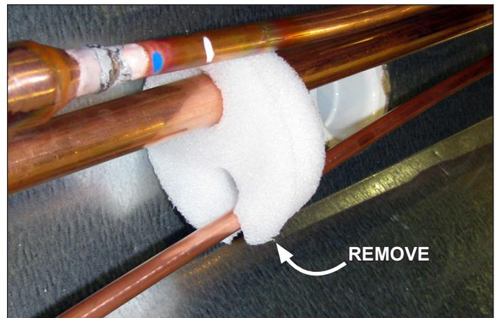
Fig. 11 Remove the shipping blocks
