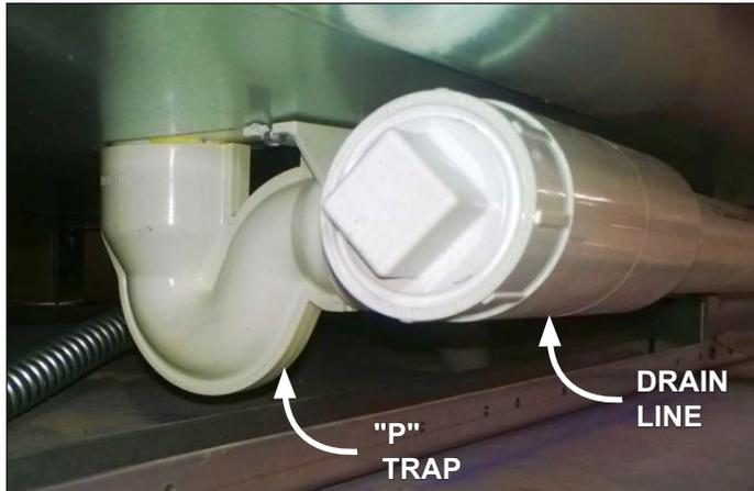
Fig. 12 “P” trap; drain line
