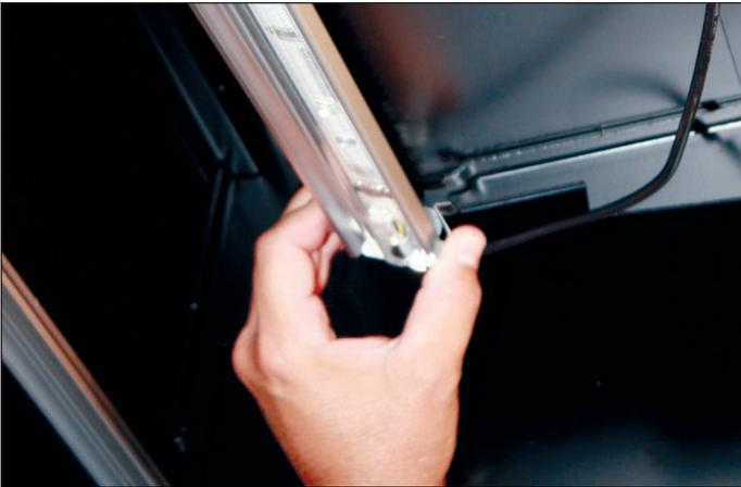
**Fig. 20** Remove the old LED luminaire
