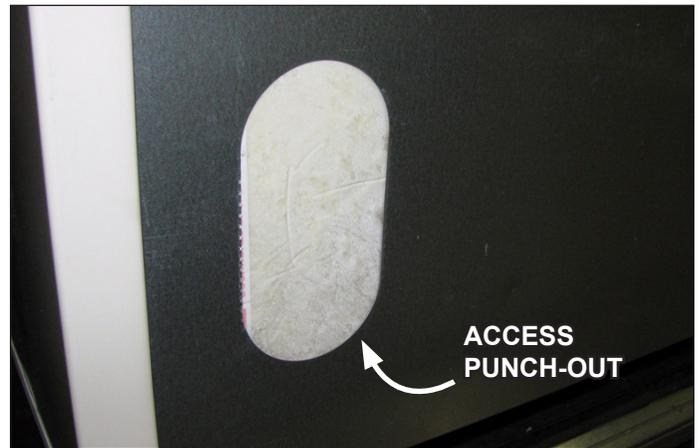
Fig. 10 Penetrate foam as needed to access piping
