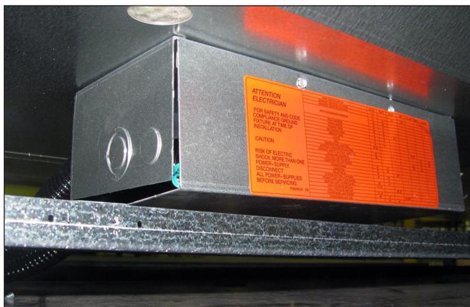
Fig. 13 Junction box beneath case
