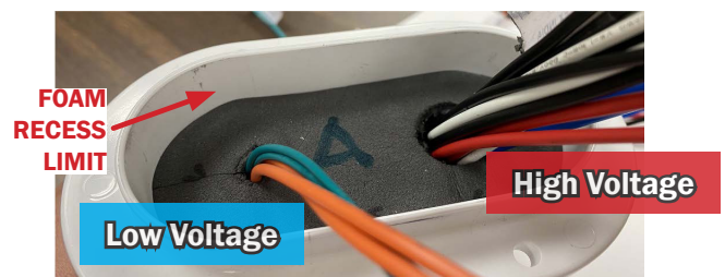
Fig. 58 Foam recess limit: 3/4" below egress opening
