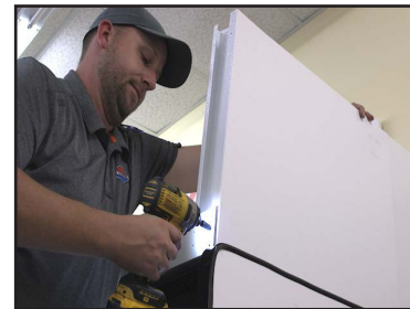
Fig. 86 Secure end panel to front fascia
