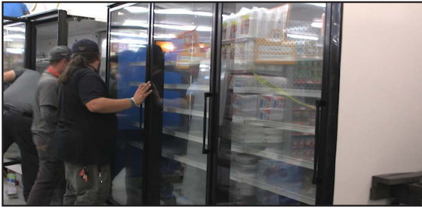
Fig. 51 Push second case close to first case
