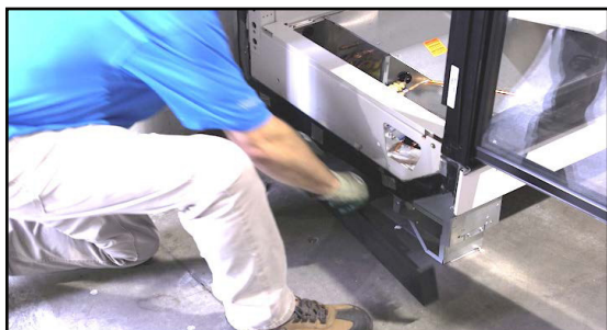
Fig. 76 End kickplate installation
