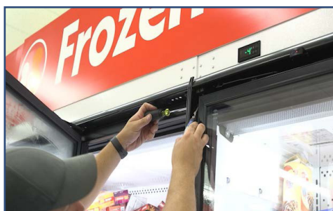
Fig. 91 Install frame trim between doors
