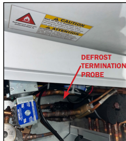
Fig. 103 LT defrost termination probe sensor location
