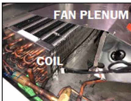
Fig. 105 Coil & single-piece fan plenum
