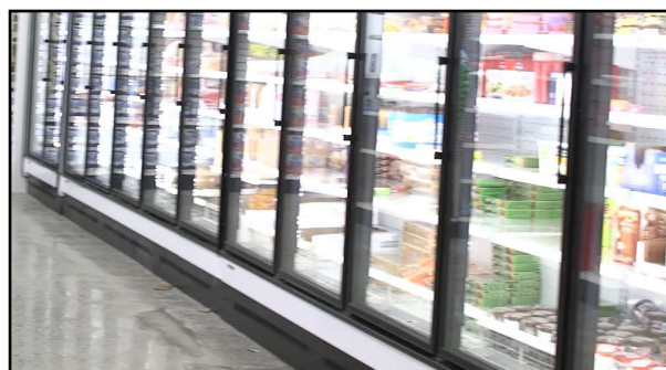
Fig. 80 Case lineup with kickplates installed
