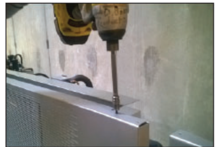
Fig. 3 Attach the front fascia to the recessed coil shroud.
