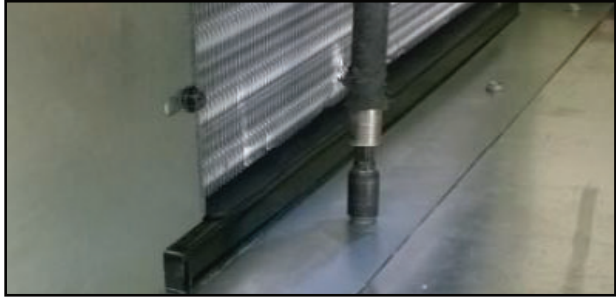
Retrieve shipped-loose intake guard from inside case. Nest top edge into "V" retainer flange at top of air-block. Fasten bottom to case.
