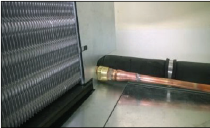
Retrieve shipped-loose condensing unit air-block from inside case. Match cut outs to condensing unit and fasten by backing out and re-installing screws from the condenser coil.
