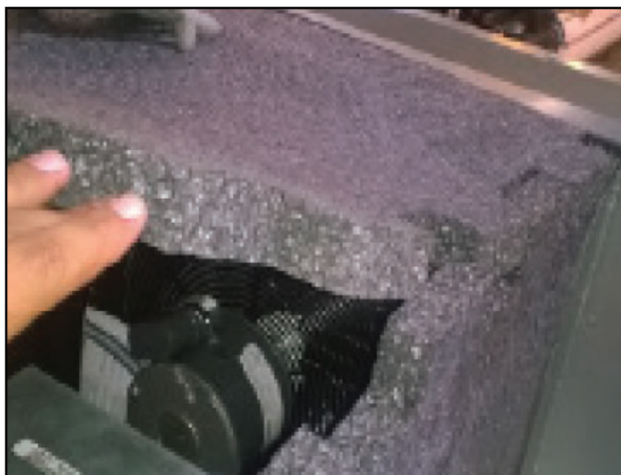
Top panel installs under metal edge, filling in the pre-cut slots.
