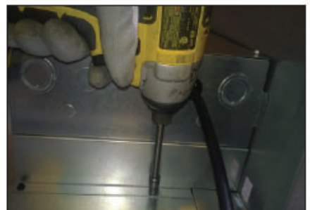
Fig. 6 Secure electrical box to case body.
