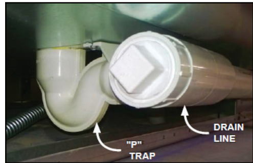
Fig. 7 “P” trap; drain line
