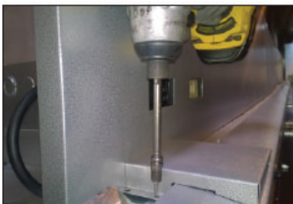
Fig. 7 Install heater wire cover.
