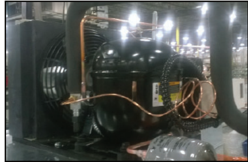
Fig. 6 Condensing unit on top of case
