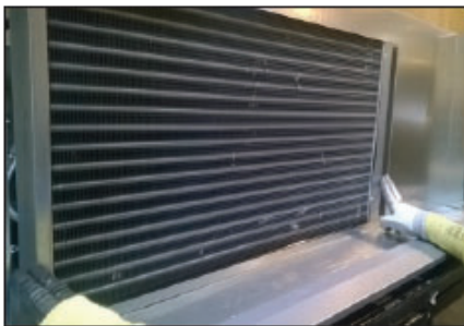
Fig. 1 Install recessed coil shroud.
