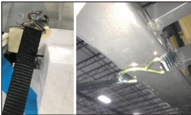
Connect ratchet strap from the top to the bottom.
