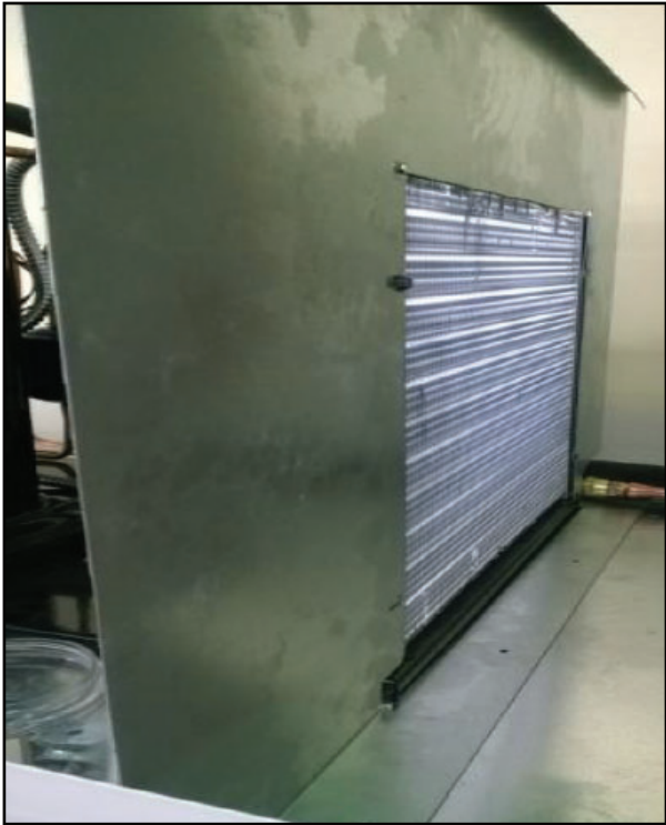
Retrieve shipped-loose condensing unit air-block from inside case. Match cut outs to condensing unit and fasten by backing out and re-installing screws from the condenser coil.
