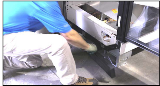
Fig. 74 End kickplate installation
