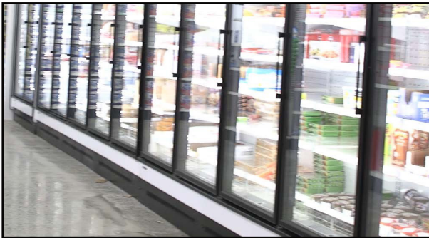
Fig. 78 Case lineup with kickplates installed
