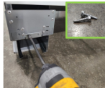
Fig. 39 Fasten locator lip
