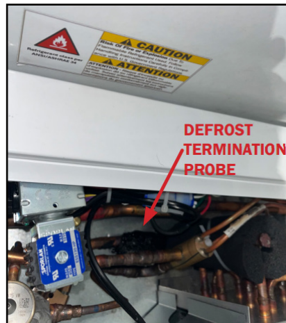
Fig. 102 LT defrost termination probe sensor location
