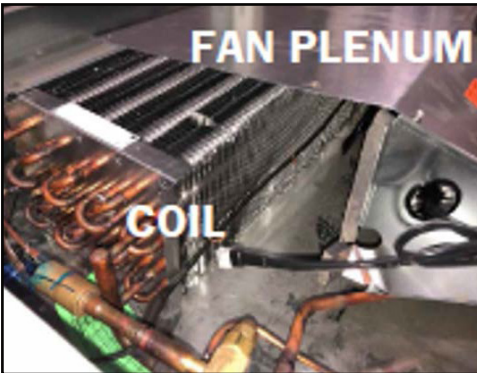
Fig. 104 Coil & single-piece fan plenum
