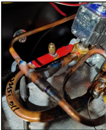
Fig. 106 Schrader port locations
