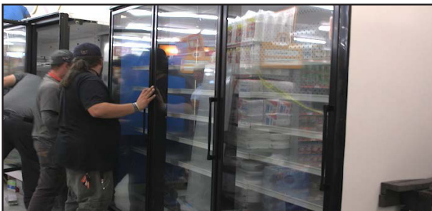
Fig. 43 Push second case close to first case
