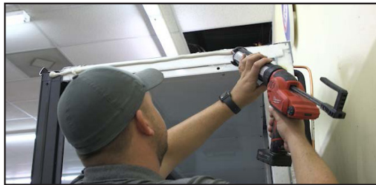
Fig. 42 Apply Sealant (Low Temp)
