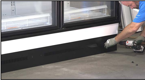
Fig. 77 Secure the kickplate to base frame
