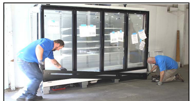
Fig. 76 Insert kickplate's top flange behind front panel
