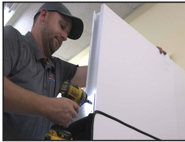
Fig. 84 Secure end panel to front fascia
