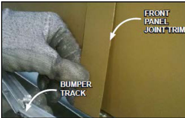
Fig. 66 Front panel trim installed behind bumper tracks
