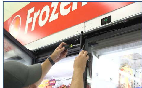
Fig. 89 Install frame trim between doors
