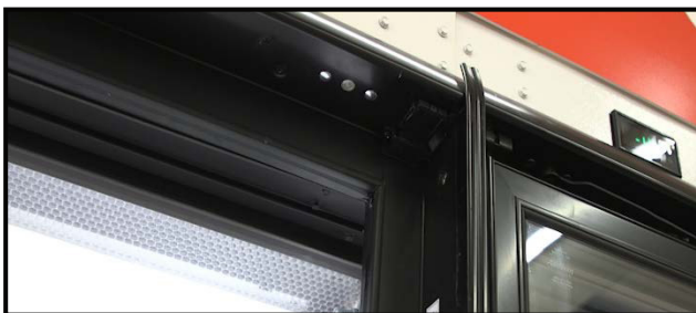
Fig. 73 Door frame trim installed
