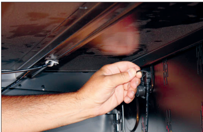
Fig. 24 Unplug the LED luminaire
