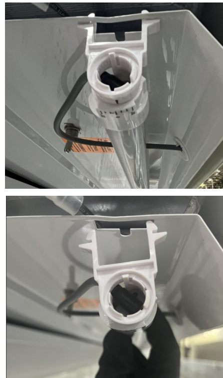
Fig. 26 Squeeze the latching clips and pull the luminaire free
