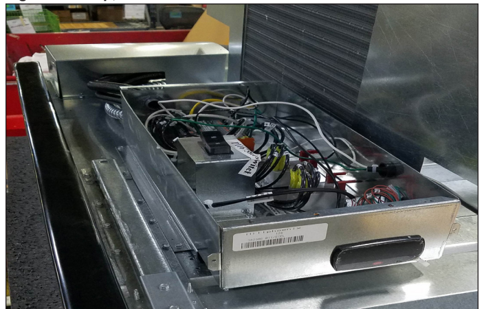
Fig. 14 Electrical junction box on top of case
