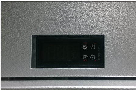
Fig. 7 Carel controller visible through cut-out in front fascia.
