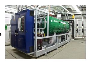
The materials and components of CO<sub>2</sub> systems operate safely and efficiently at elevated pressure. Higher pressure may provide more volume of heat for heat reclamation and subsequent use elsewhere in the facility, resulting in energy cost savings.
