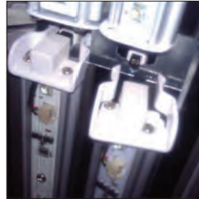
1. Squeeze plastic clips at one end, pinch the latching clips and pull the luminaires free.
