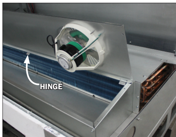
Fig. 15 Pressure plate and hinges (underside)
