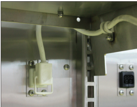
Fig. 4 T-8 light power cord (WHITE)
