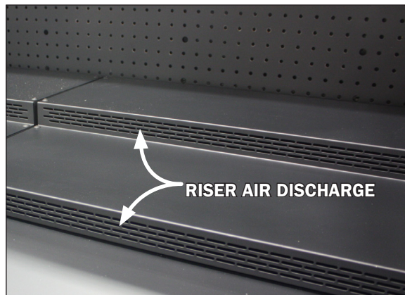
Fig. 21 Step riser perforated front air discharge
