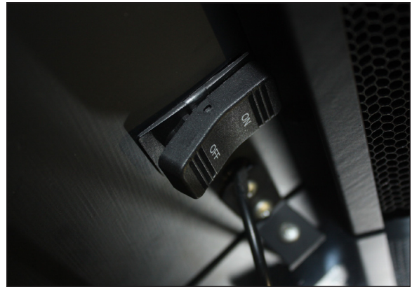
Fig. 12 Upper cornice light switch
