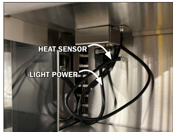
Fig. 7 LED light power cord & heat sensor
