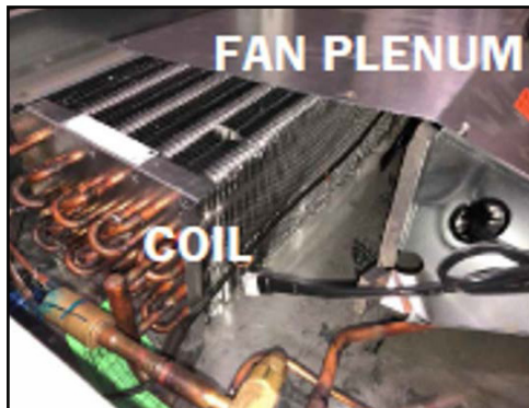
Fig. 102 Coil & single-piece fan plenum
