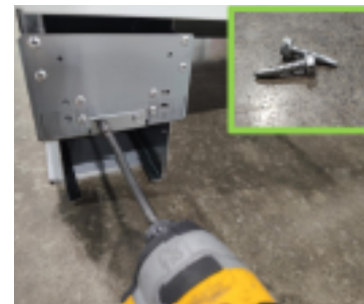
Fig. 39 Fasten locator lip
