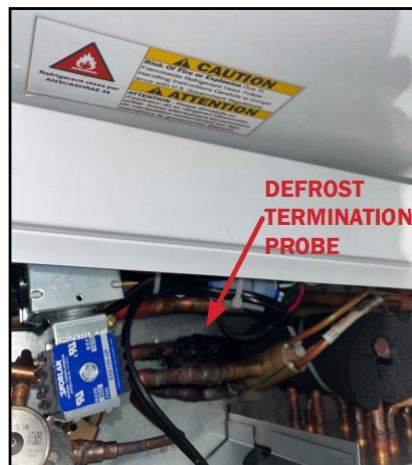
Fig. 100 LT defrost termination probe sensor location
