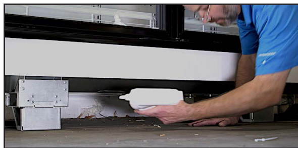
Fig. 49 PVC drain oriented left toward grease trap.
