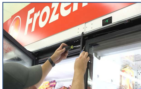
Fig. 89 Install frame trim between doors
