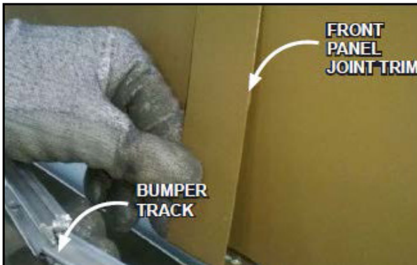
Fig. 66 Front panel trim installed behind bumper tracks
