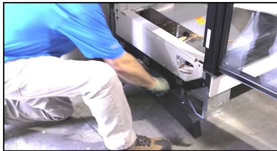
Fig. 74 End kickplate installation
