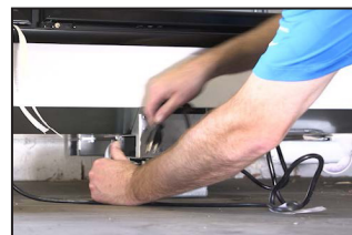
Fig. 51 Plug pump into pump receptacle
