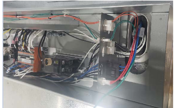
Fig. 59 Connect harnesses to their mates inside junction box
