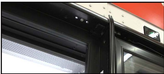
Fig. 73 Door frame trim installed
