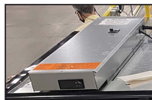
Fig. 92 Switch location on junction box
