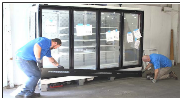
Fig. 76 Insert kickplate's top flange behind front panel
