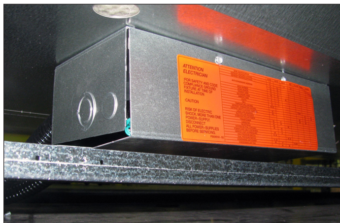
Fig. 8 Junction box beneath case
