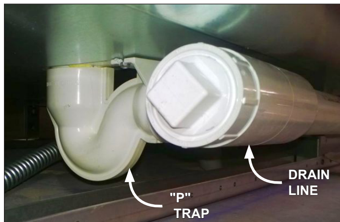
Fig. 7 “P” trap; drain line
