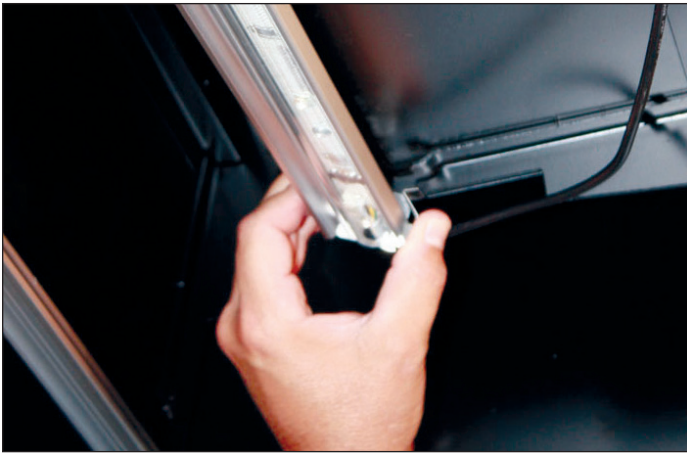
Fig. 12 Remove the old LED luminaire
