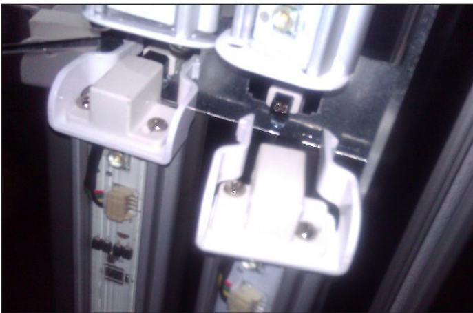
Fig. 13 Squeeze the latching clips and pull the luminaire free
