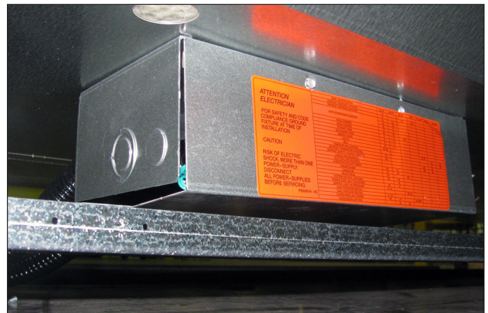
Fig. 11 Junction box beneath case
