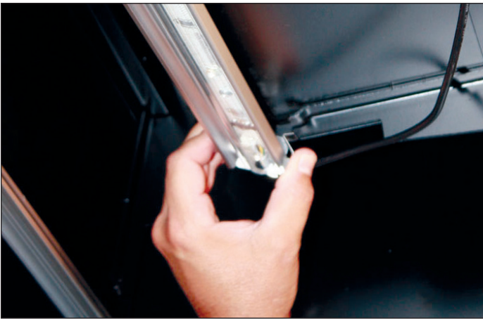
Fig. 15 Remove the old LED luminaire
