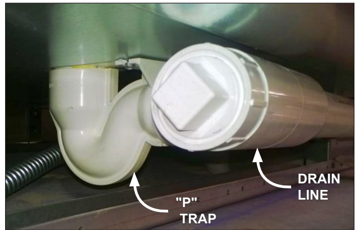
Fig. 10 “P” trap; drain line
