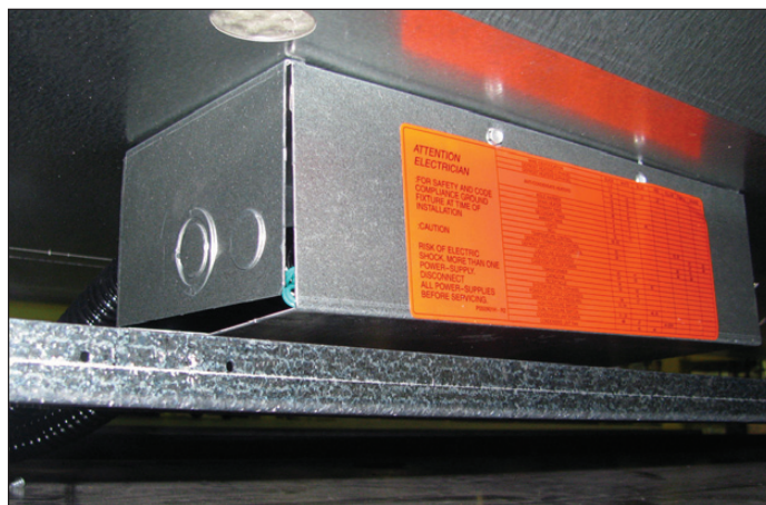
Fig. 11 Junction box beneath case
