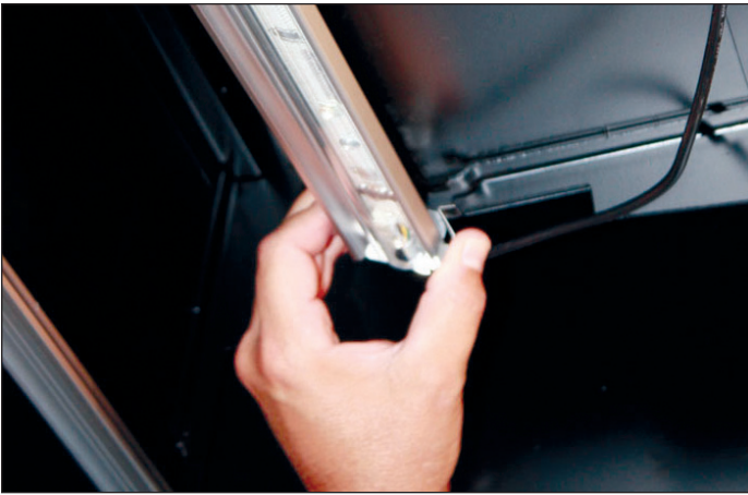
Fig. 15 Remove the old LED luminaire
