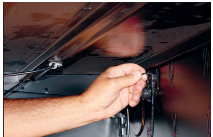
Fig. 14 Unplug the LED luminaire
