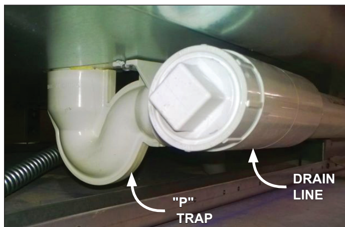
Fig. 10 “P” trap; drain line
