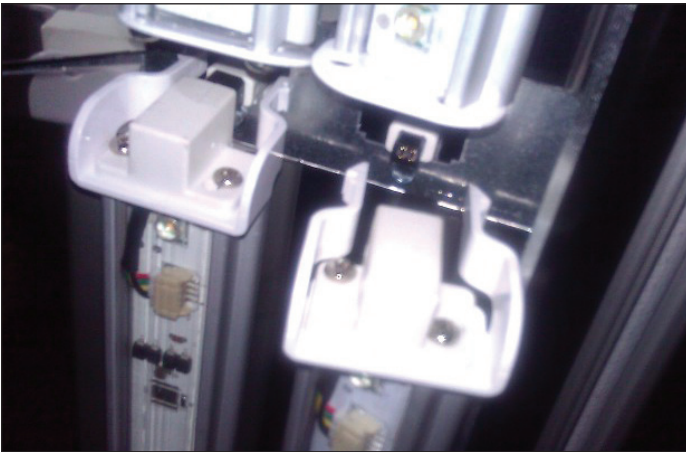
Fig. 16 Squeeze the latching clips and pull the luminaire free
