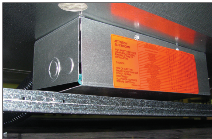
Fig. 13 Junction box beneath case
