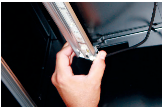
Fig. 11 Remove the old LED luminaire
