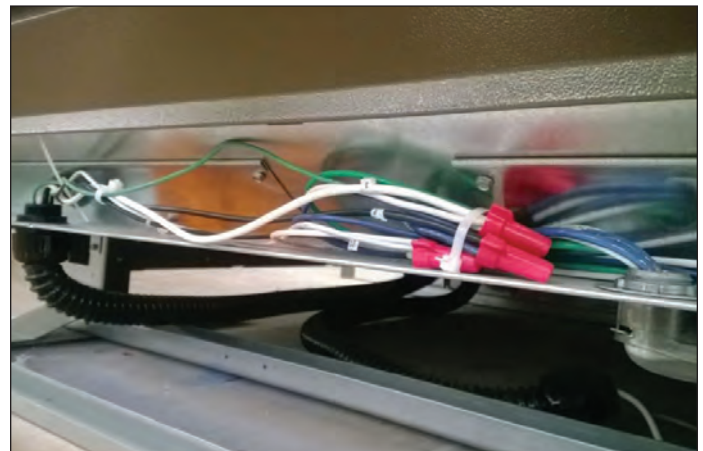
Fig. 7 Raceway electrical wiring
