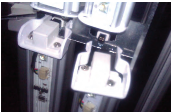
Fig. 12 Squeeze the latching clips and pull the luminaire free
