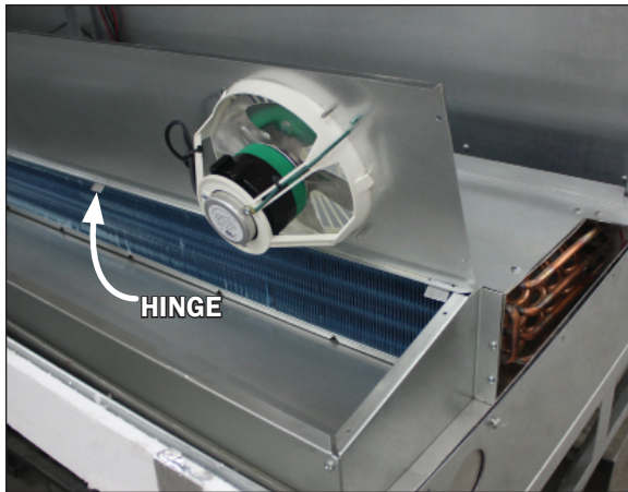
Fig. 15 Pressure plate and hinges (underside)
