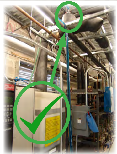
Needed vent properly installed
