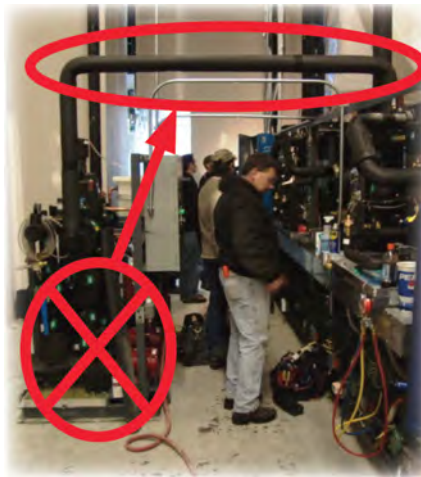
Needed vent not installed
