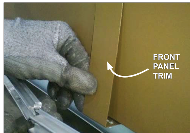
Fig. 5 Front panel joint trim
