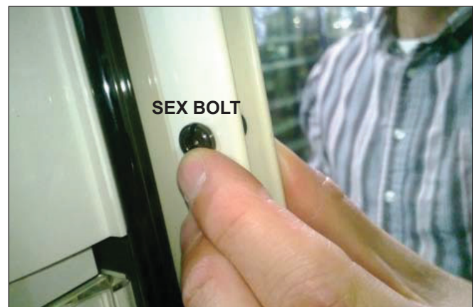
Fig. 6 Sex bolts for closing case frame gap
