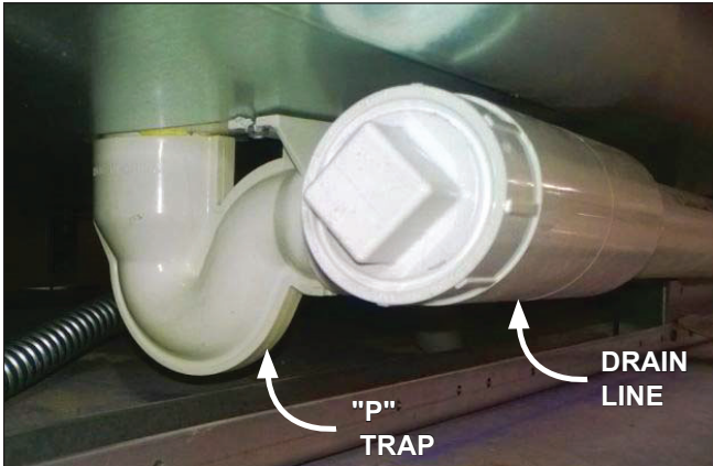
Fig. 11 “P” trap; drain line
