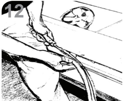
Insert the nose bumper into the master bumper channel. Roll nose bumper into channel along entire lineup (up to 96'). We recommend that the nose bumper be left in the store 24 hours before installing. DO NOT STRETCH THE BUMPER during installation as it will shrink to its original length and leave a gap.
