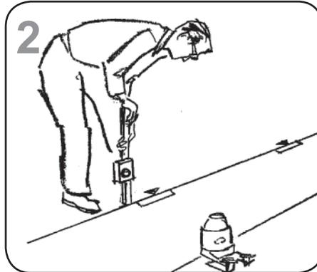
Leveling is necessary to ensure proper case alignment. Locate the highest point on the chalk line as a reference for determining the height of shim-pack levelers. A laser transit is recommended for precision and requires just one person.
