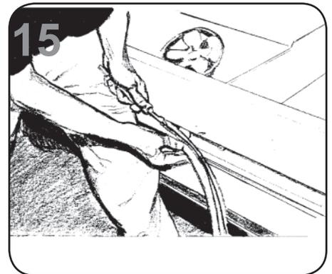
Insert the nose bumper into the master bumper channel. Roll the nose bumper into the channel along entire lineup (up to 96'). We recommend that the nose bumper be left in the store 24 hours before installing. DO NOT STRETCH the bumper during installation, as it will shrink to its original length and leave a gap.
