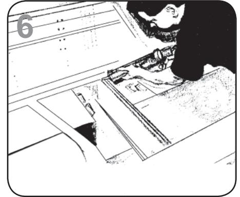
6 Seal the joints along the pipe chase seam with the caulk provided.
