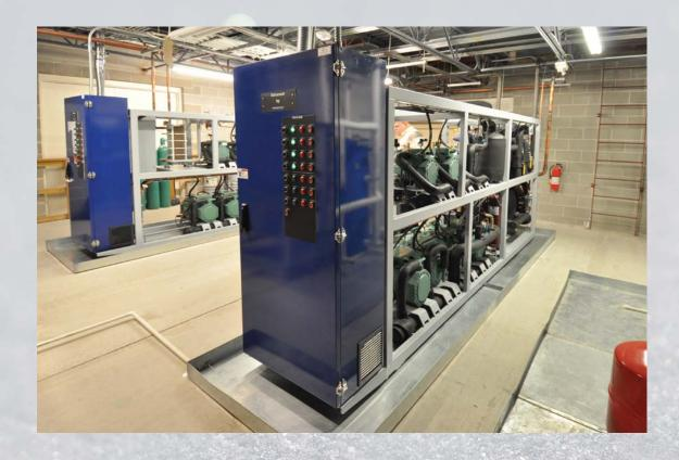
The Hillphoenix<sup>®</sup> Advansor  $CO_2$  booster system is a member of our sustainable line of refrigeration systems. The Advansor  $CO_2$  booster system is an HFC-free refrigeration alternative that utilizes carbon dioxide as the only refrigerant in the system. Hillphoenix customers can take advantage of the inherent benefits of  $CO_2$  and combine them with those of other Second Nature systems - reducing direct refrigerant emissions to the lowest level possible.
