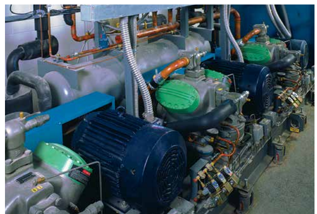
Open drive compressors are just one of the many compressor choices you have
