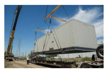
Delivered complete from the factory preassembled, piped, wired and tested.
