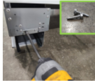
Now fasten the locator lip with 8-size Tek screws provided.
