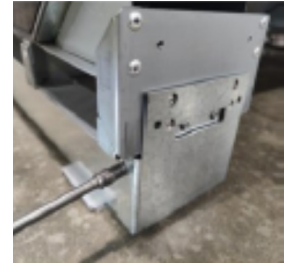
Place front fastening Plates over Side Fastening Holes; fasten plate with Tek screws on each side.
