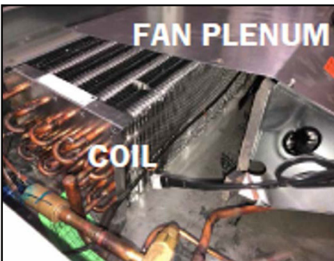
Coil & single-piece fan plenum
