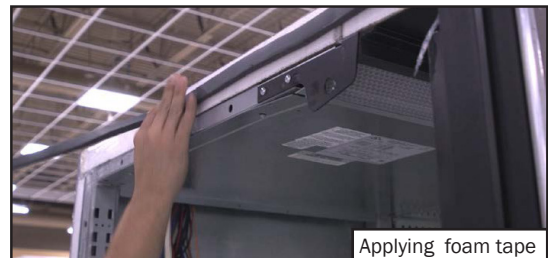
Applying foam tape
