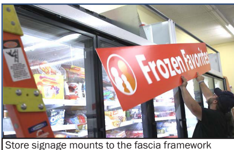
Check the vertical alignment of the panel and adjust if necessary
