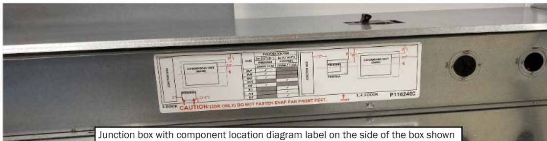
Junction box with component location diagram label on the side of the box shown
