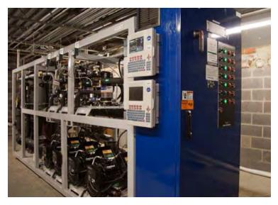
CO<sub>2</sub>-based, air-cooled system could operate efficiently in locations where outdoor ambient temperatures were above 80° F. This climate-driven limitation was dubbed the "CO<sub>2</sub> Equator", which referred to the generally accepted geographical limit for cost-effective deployment of CO<sub>2</sub> systems in food retail.
