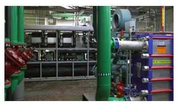
subsequently captured. The resulting heat reclaim adds to the list of benefits that CO2 can provide and that users in other applications, ranging from supermarkets to ice rinks, can likewise take advantage of.
