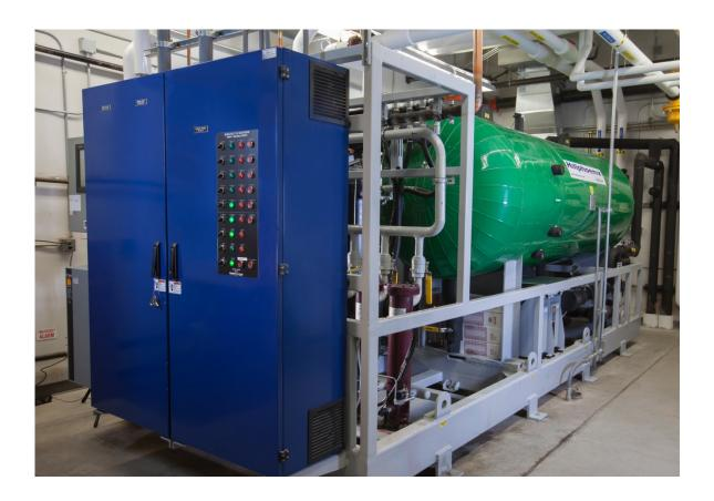
The Hillphoenix® Advansor system provides a much higher coefficient of performance (COP) than that of ammonia-calcium chloride systems. And easily accessible heat recovery can be a heating source for the entire facility including indoor areas, locker rooms, and utility water.
